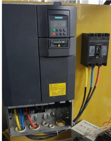
Fig. 5.17 Siemens Micromaster 440 of 22kW variable frequency drive
